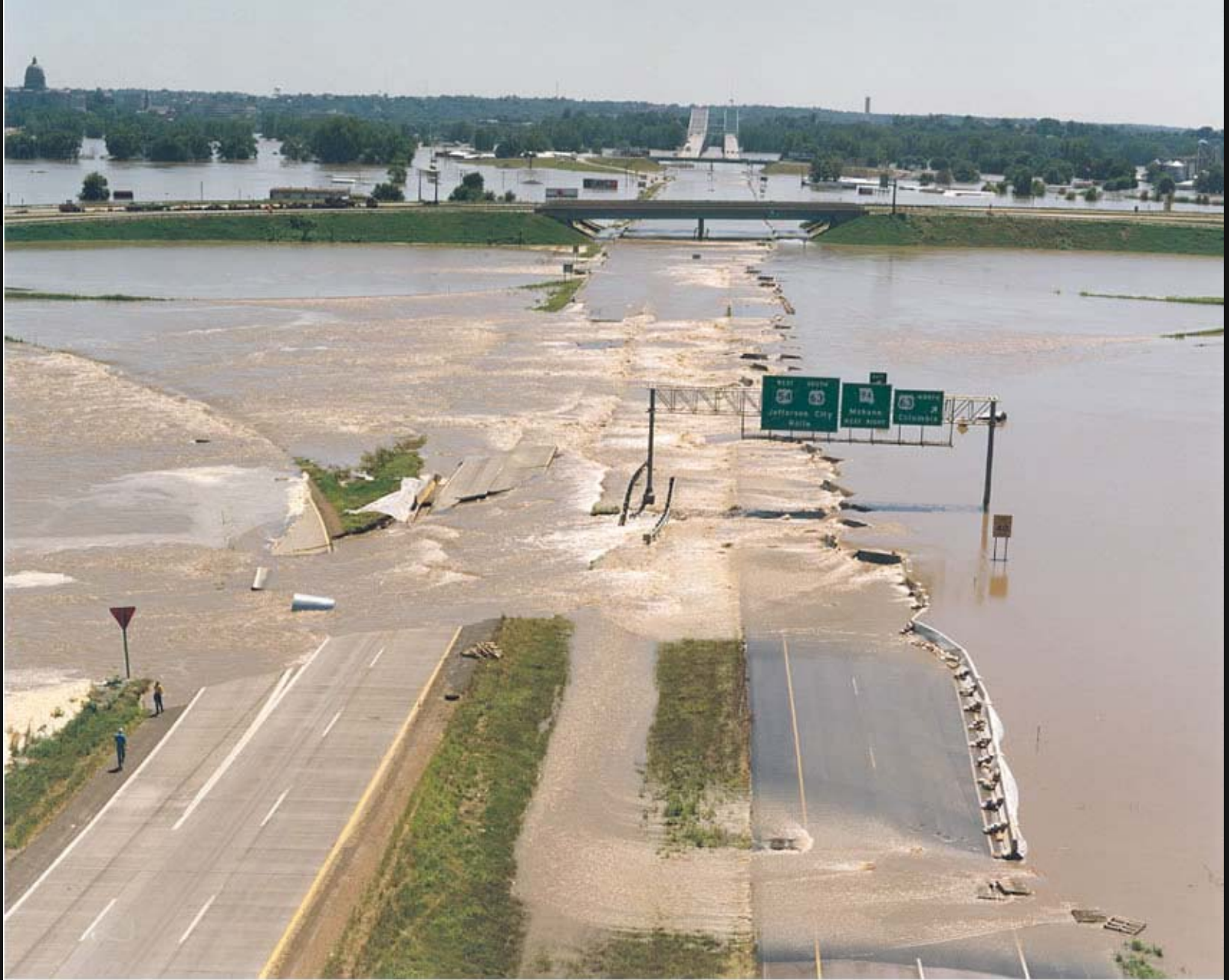
Aerial view of the Missouri River flooding on July 30, 1993, at U.S. Highway 54 just north of Jefferson City, Missouri, looking south (photograph from the Missouri Highway and Transportation Department).
