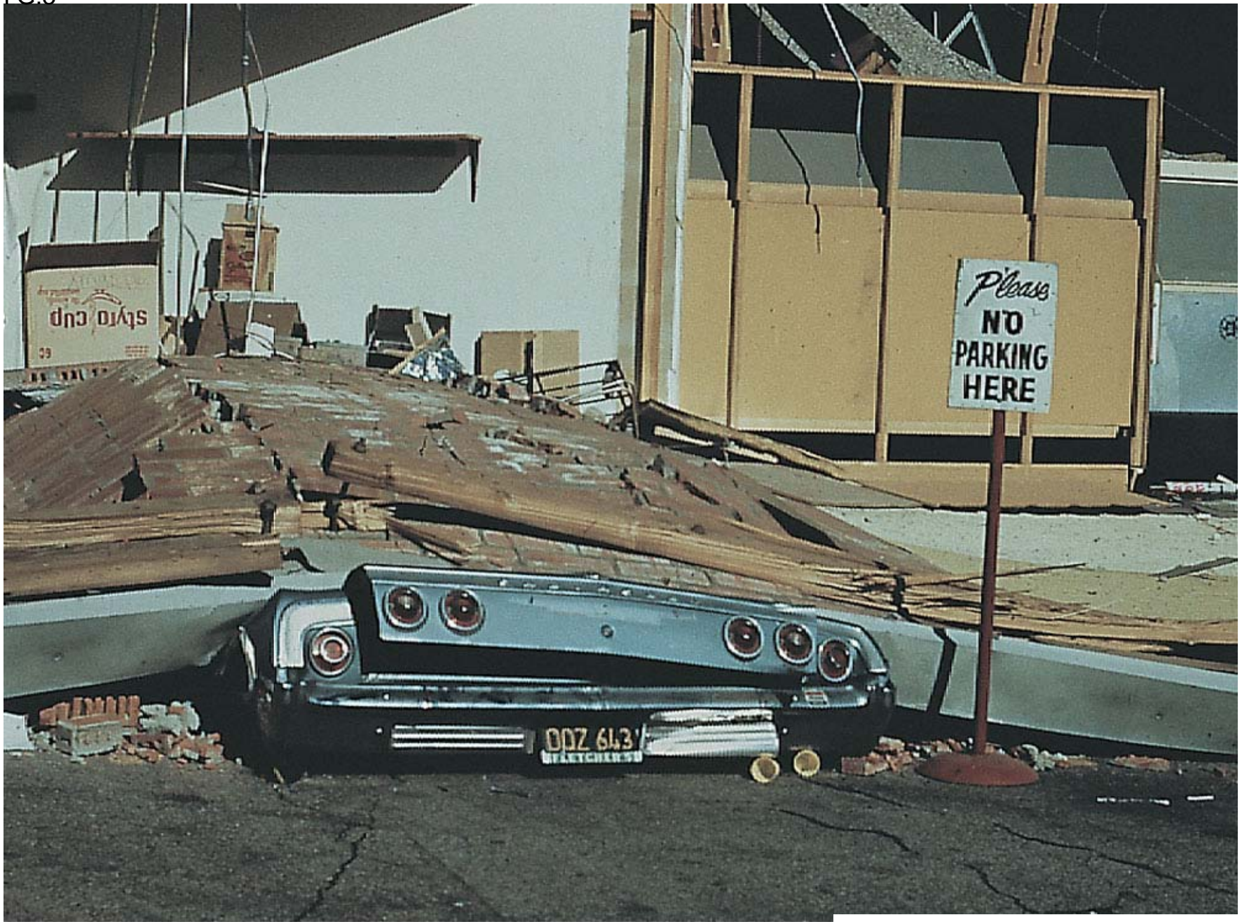
Damage from the 1971 San Fernando Valley, CA earthquake
