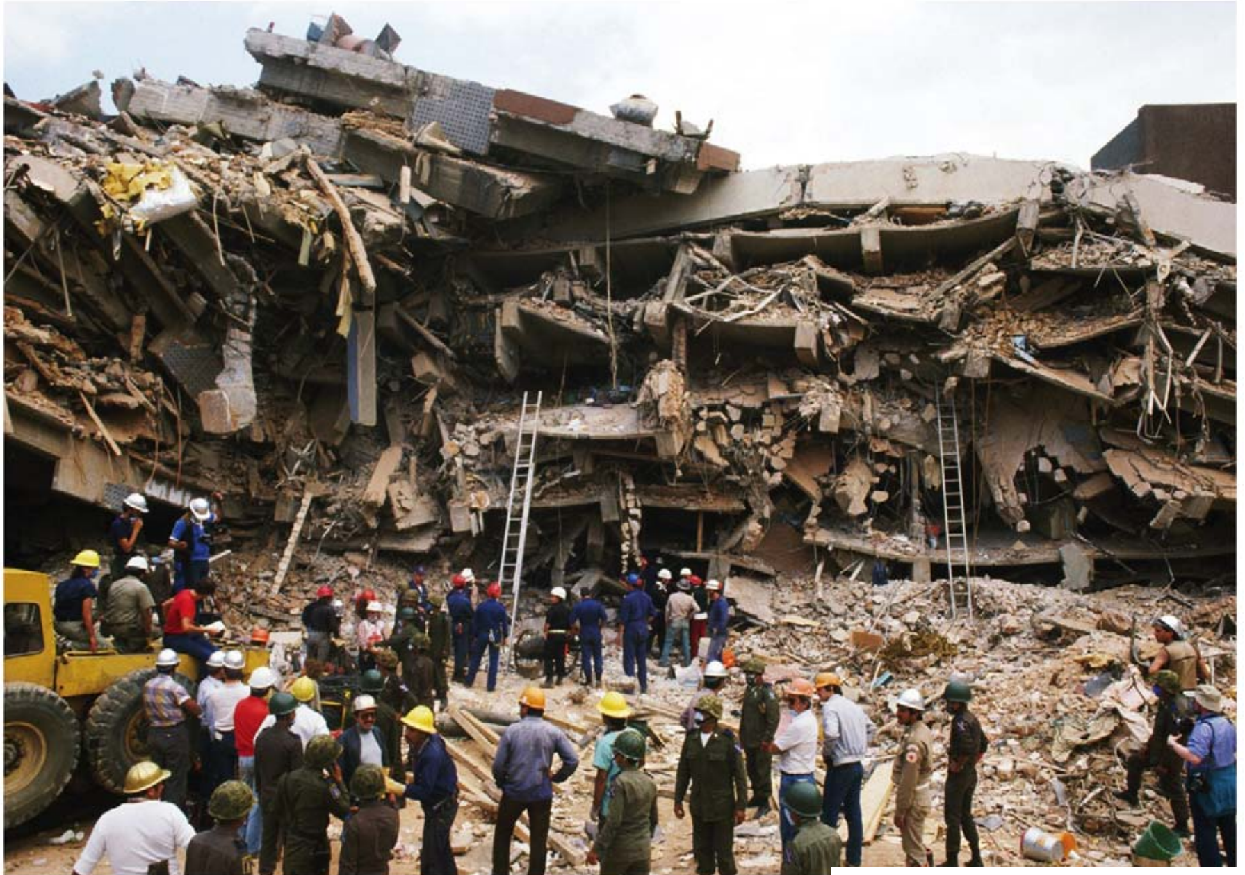
1985 Mexico City earthquake (M 8.1) – damage from ground shaking
