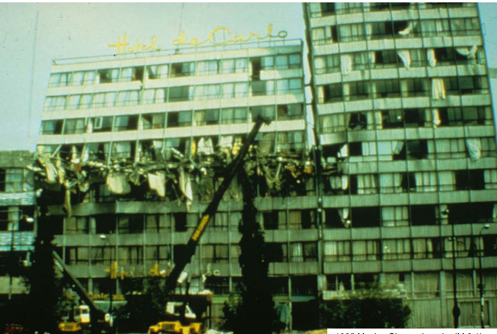
1985 Mexico City earthquake (M 8.1) – damage from ground shaking
