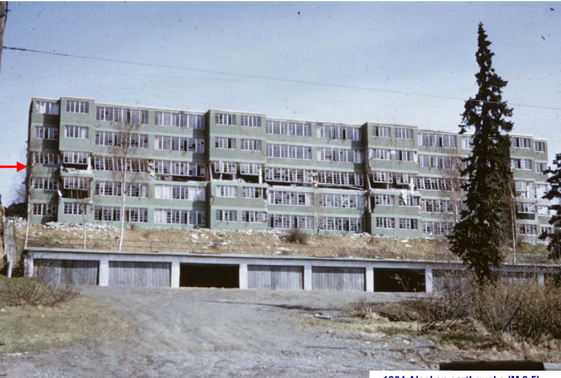
1964 Alaskan earthquake (M 8.5) – damage from ground shaking
