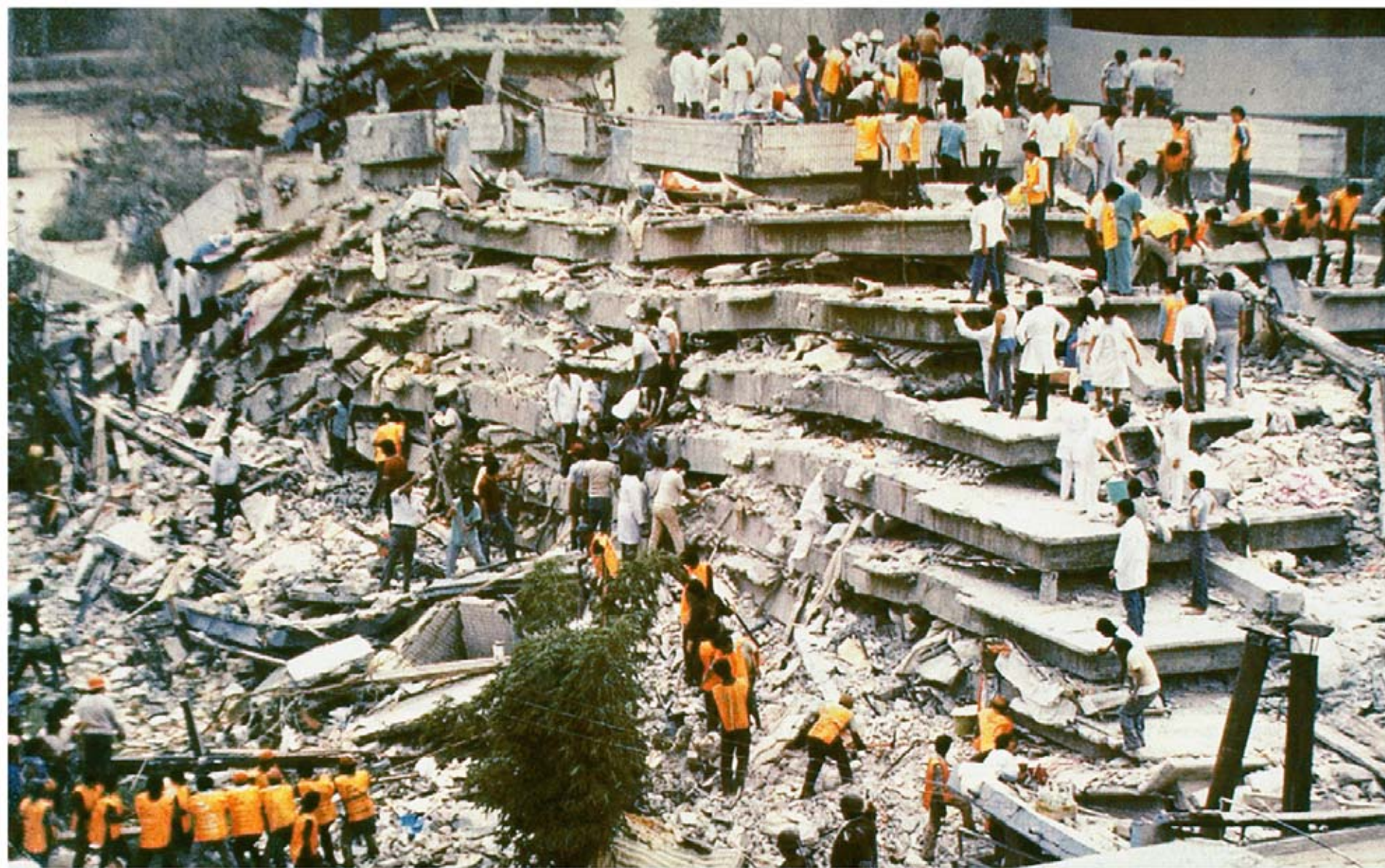
1985 Mexico City earthquake (M 8.1) – damage from ground shaking
