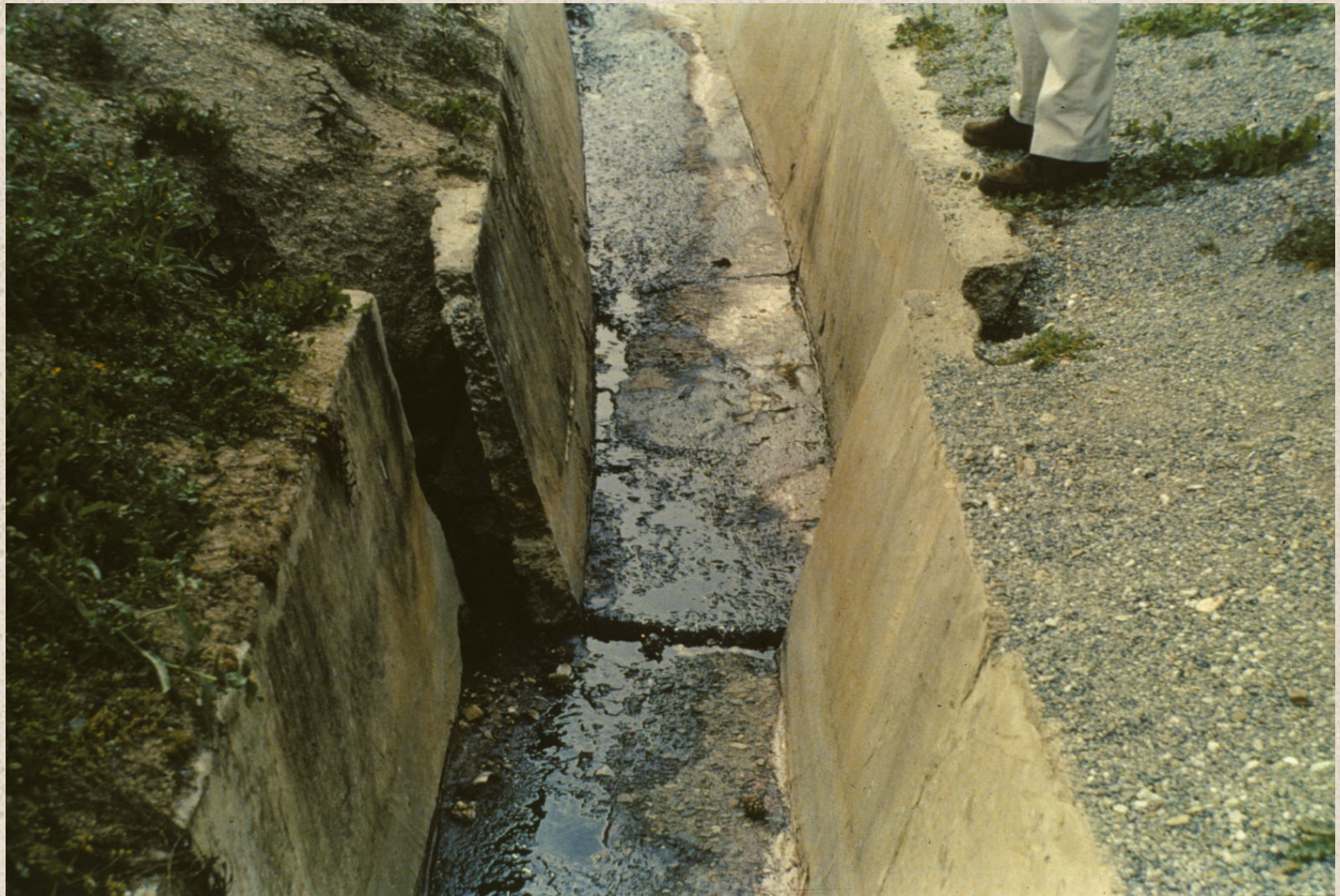
Creep along a branch of the San Andreas fault in Hollister, CA
